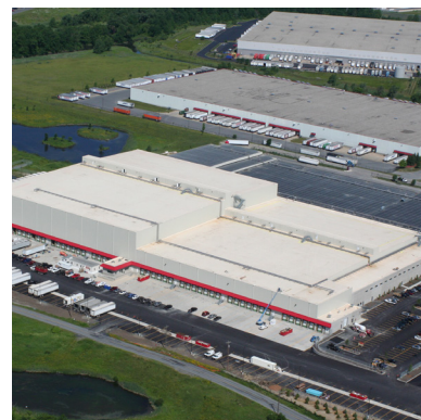
Chester, N.Y. Facility
