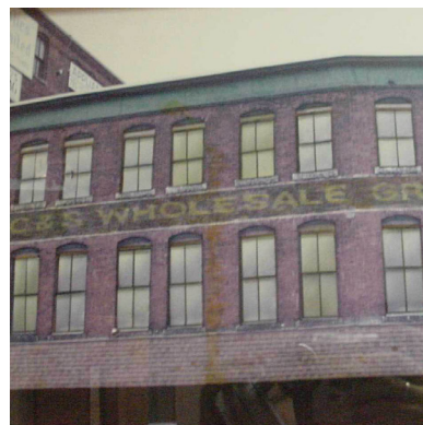
Early C&S Warehouse
